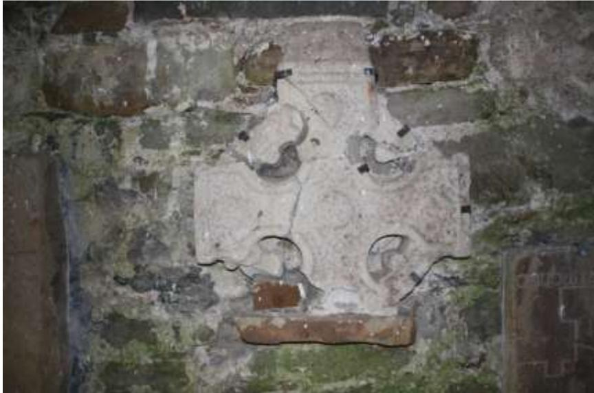
*Plate 11 Wheeled cross-head, south wall of St Caimín's Church, note breaks, metal supports, and cementitious material (C. O'Leary).*
