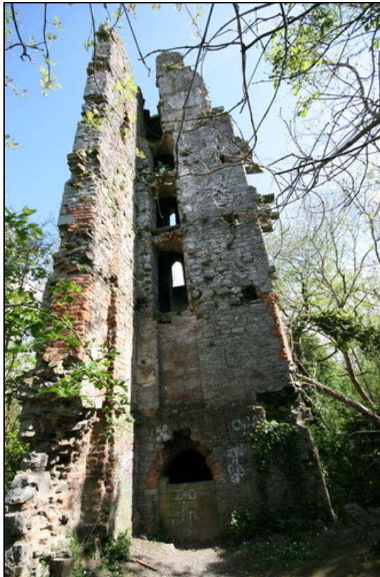
Plate 7 – AH 1/BH 26 (Plassy Mill ruins), facing south
