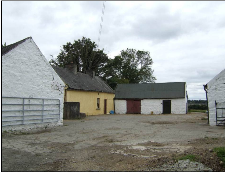
Plate 15 – BH 52 (vernacular farmyard), facing west
