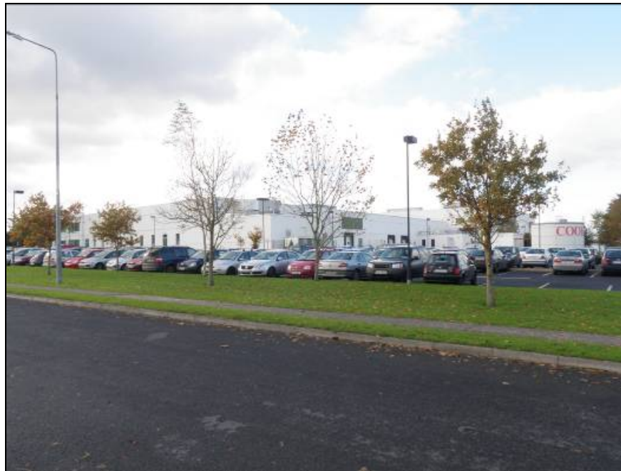
Photo 3.7.2 – COOK Ireland Facility
