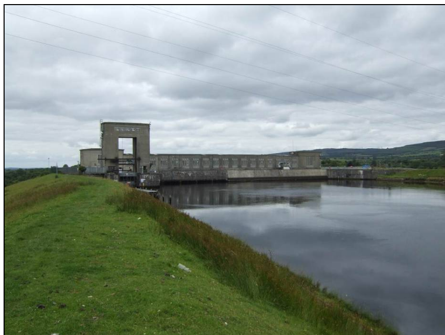
Plate 9 – BH 5 (Ardnacrusha Power Station), facing west
