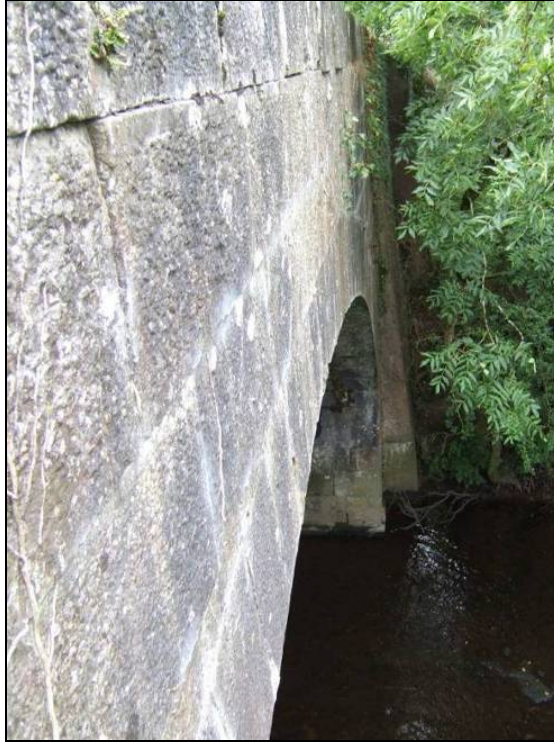
Plate 10 – BH 46 ('New Bridge'), facing southeast
