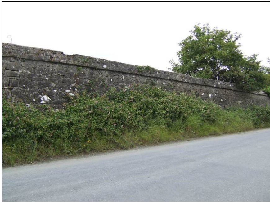
Plate 5 – BH 45 (demesne wall), facing southeast
