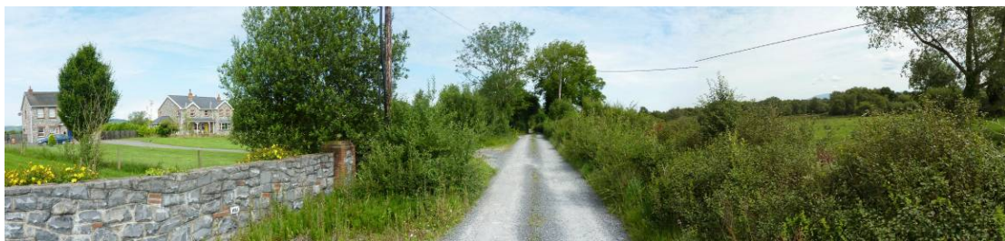
Plate 13.22: The row of houses along the lane north of Cloonoughter.
