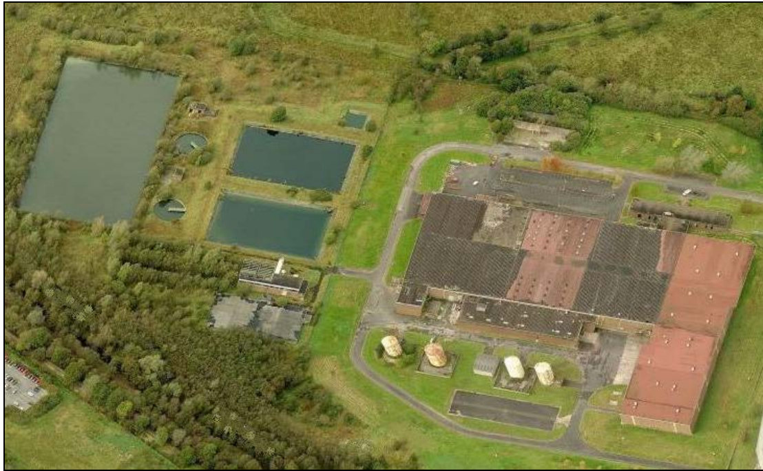
Plate 3.7.4 – Treatment Facilities, Gillogue
