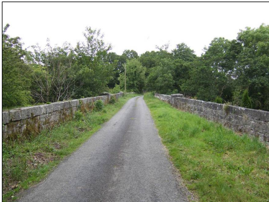
Plate 11 – The parapet walls of BH 46, facing south southwest
